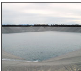
The Turley Farms lined reservoir is now about 25% full. Batter slope is 1:3.
